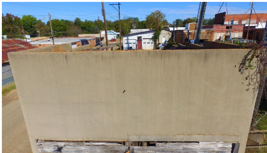
Parapet wall of the main (south) façade, with intact original stucco.
